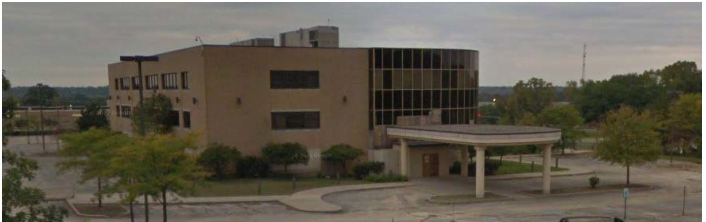
East Elevation at Main Entrance to 1300 Copperfield Avenue, Joliet, IL 60432
