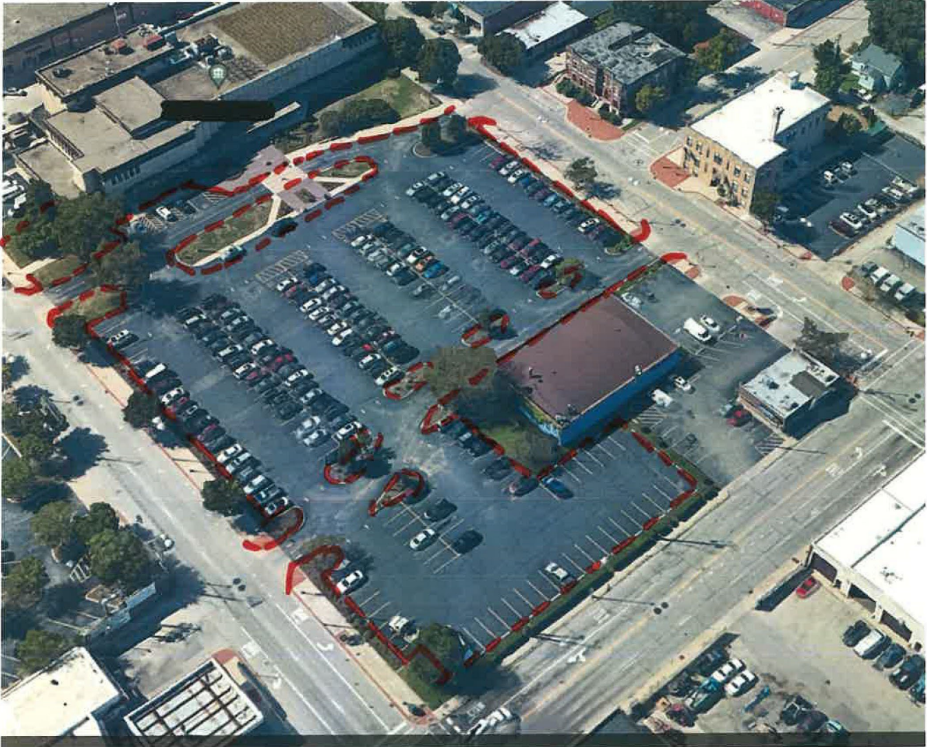
COUNY OFFICE BUILDING
