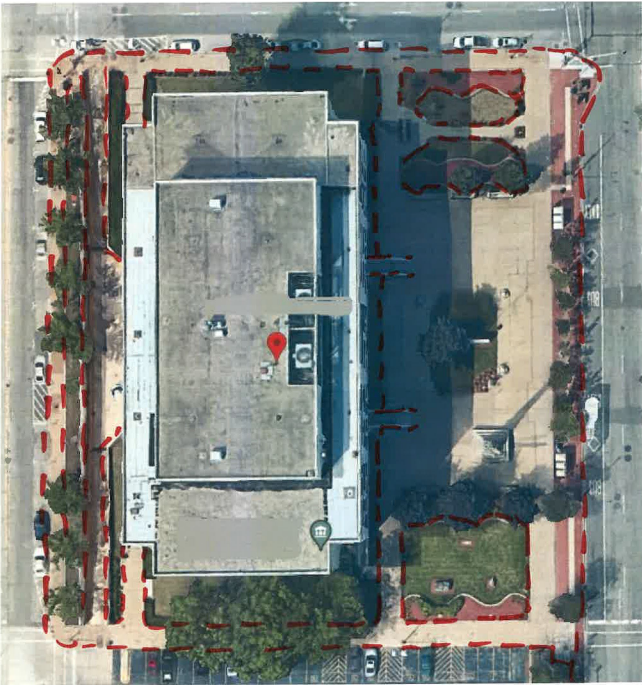
WILL COUNTY COURTYHOUSE (OLD)
