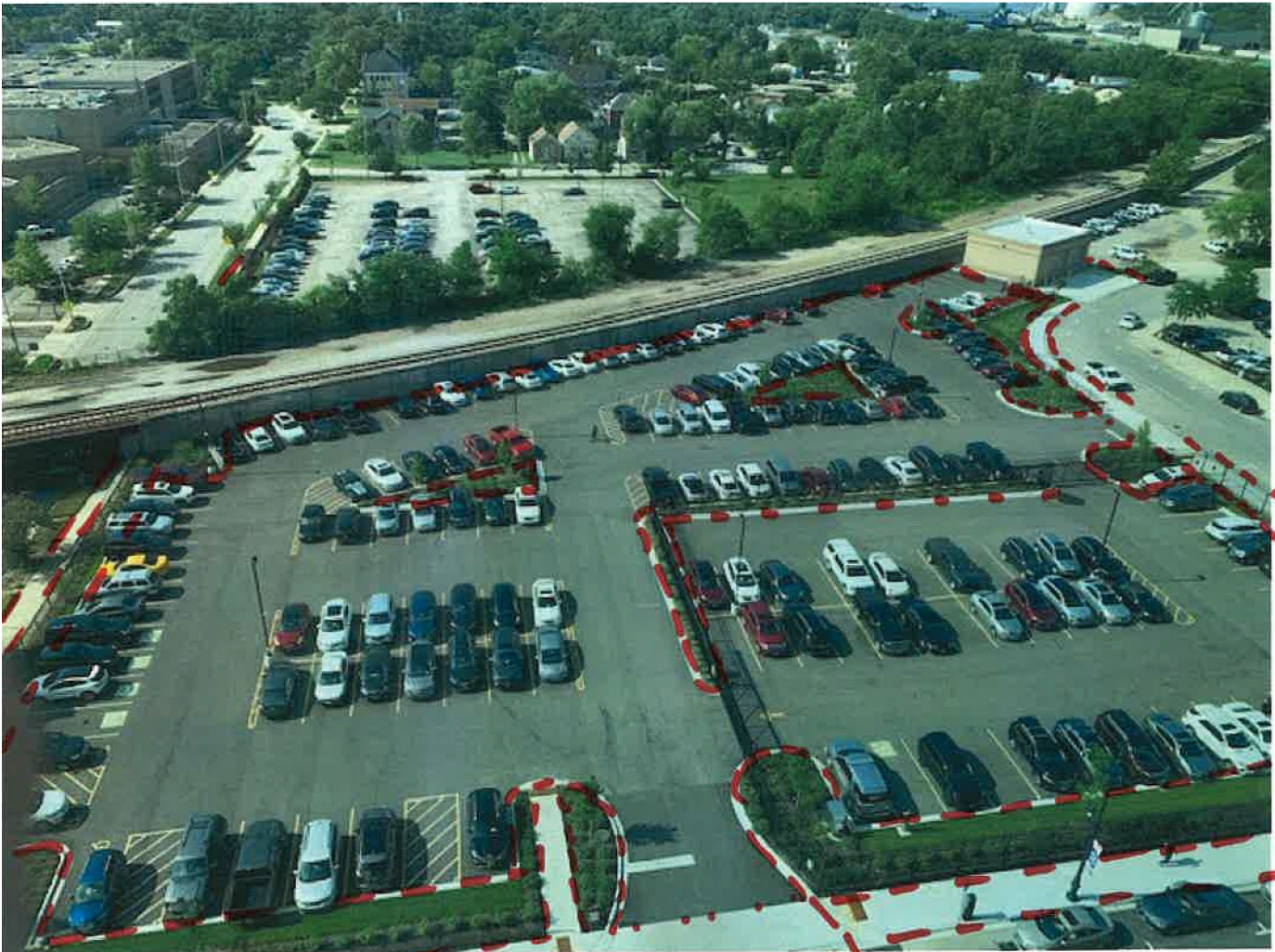
PARKING LOT A (courthouse)
