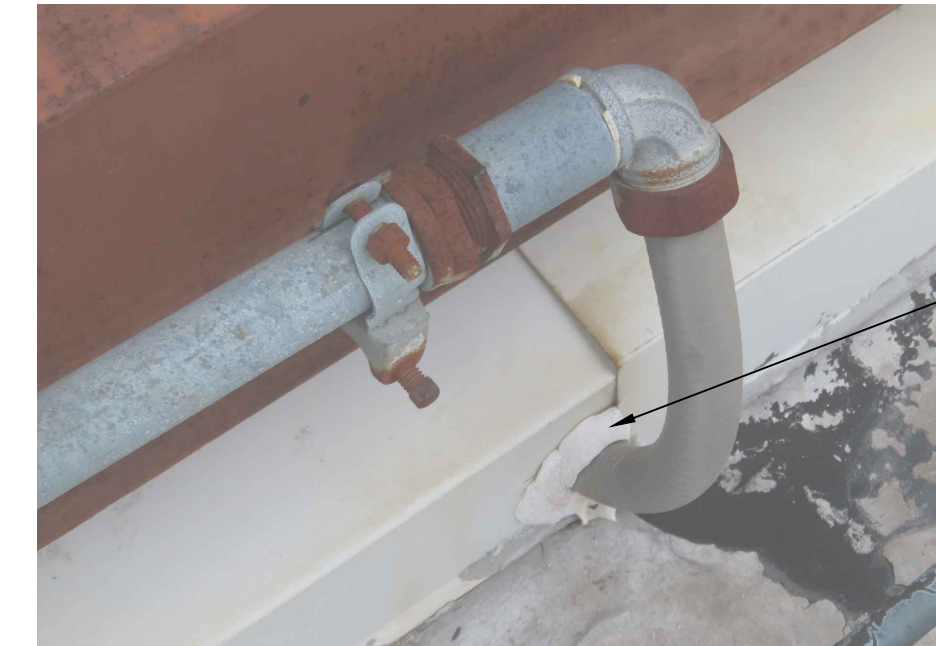
7 Conduit Through Curb Scale: Not to Scale
