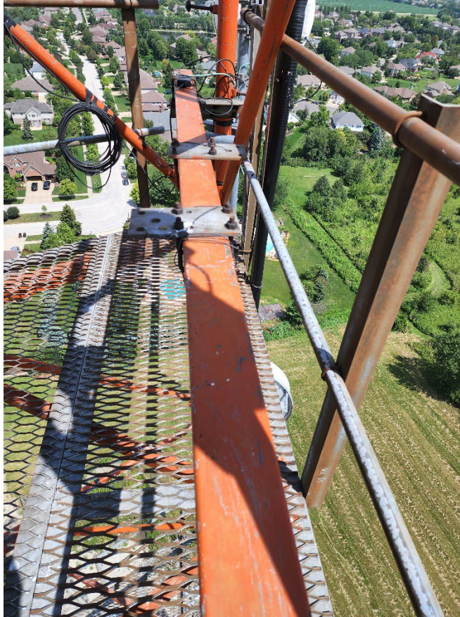
Issue 10 – removal of old equipment (mounts, tie backs, cables etc.)
