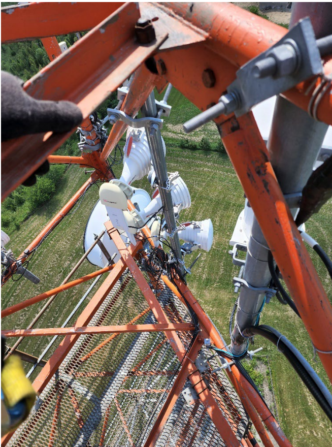
Issue 6 – wi fi clamps should be Valmont Pucks or cross over clamps
