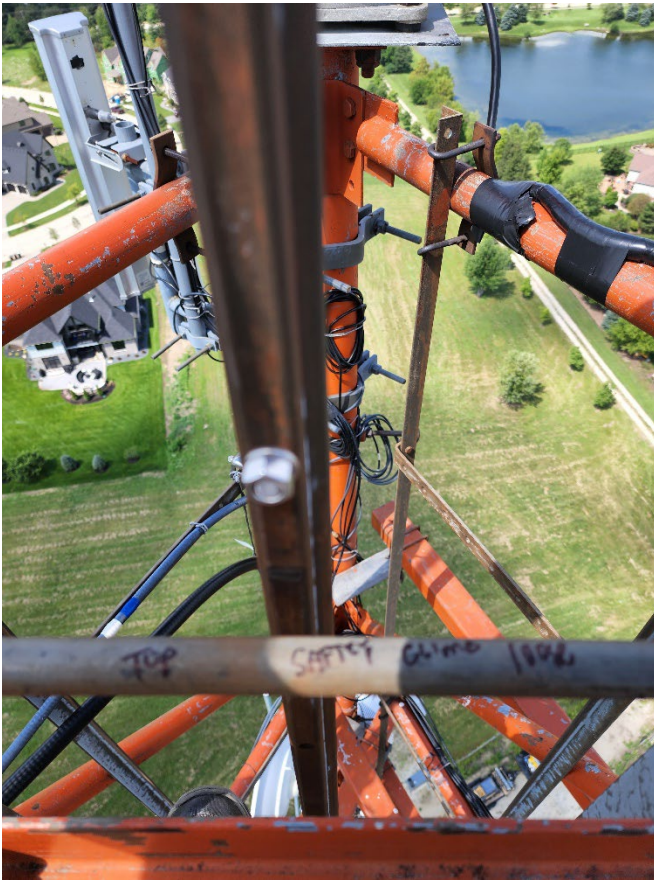
issue 1, top safety climb support missing, this is a non-standard anti climb, and we suggest replacing with a newer model
