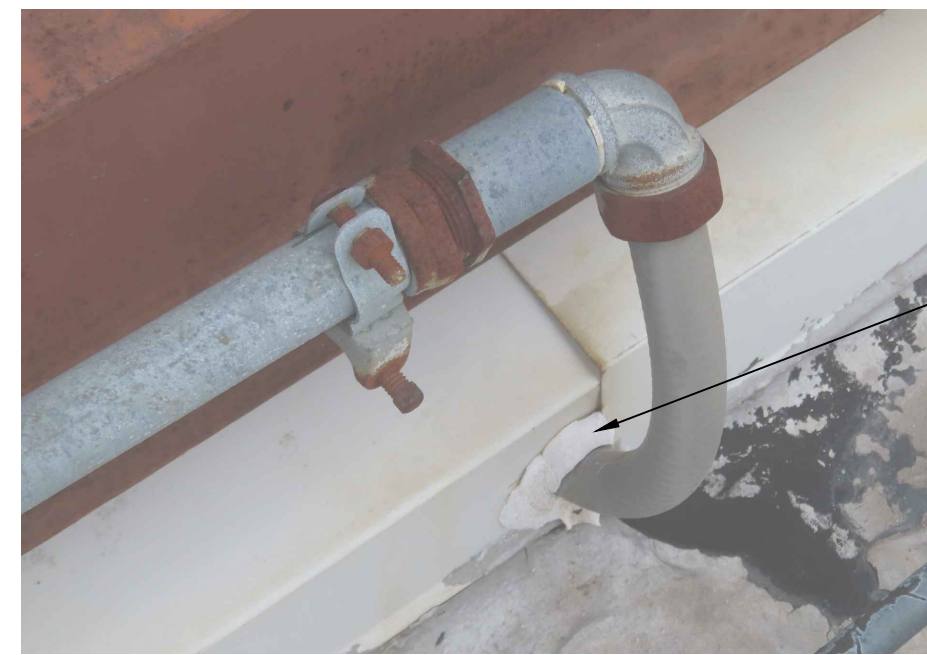
8 Conduit Through Curb Scale: Not to Scale
