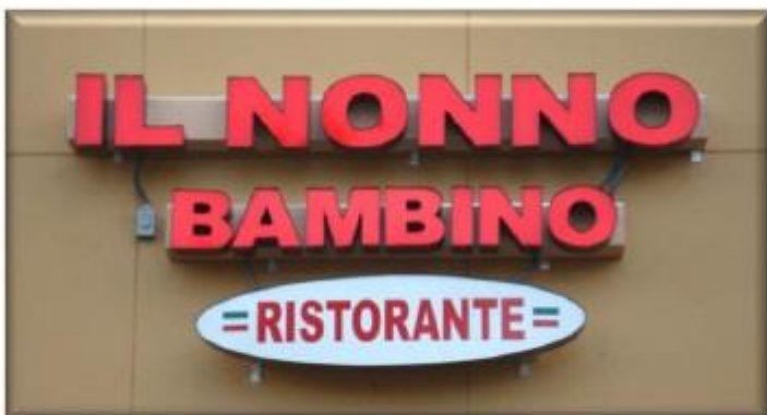
Figure 18-10: Raceway-mounted Channel Letter Sign
