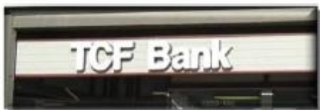
Figure 18-7: Pin-mounted Channel Letter Signs (above and below)
