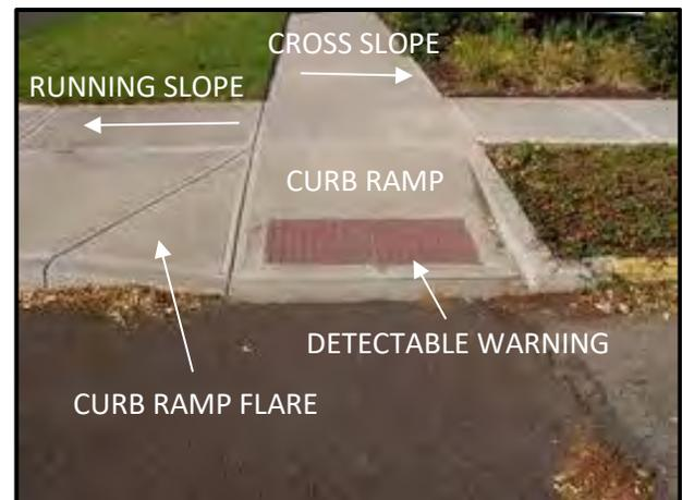
**Detectable Warning:** Surface consisting of truncated domes aligned in a square or a radial grid pattern, and built in or applied to a walking surface.
