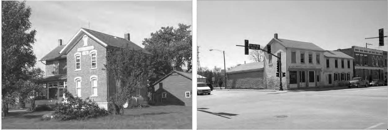
The Dague-Stewart farmhouse in Section 26 of Wheatland Township, shown above left, is a rare example of a nineteenth century brick masonry farmhouse – most of the house structures in that period were wood frame, or if built with masonry construction used local limestone. The Eagle Hotel in downtown Wilmington, shown above right, is an early example of brick masonry in an urban setting.
