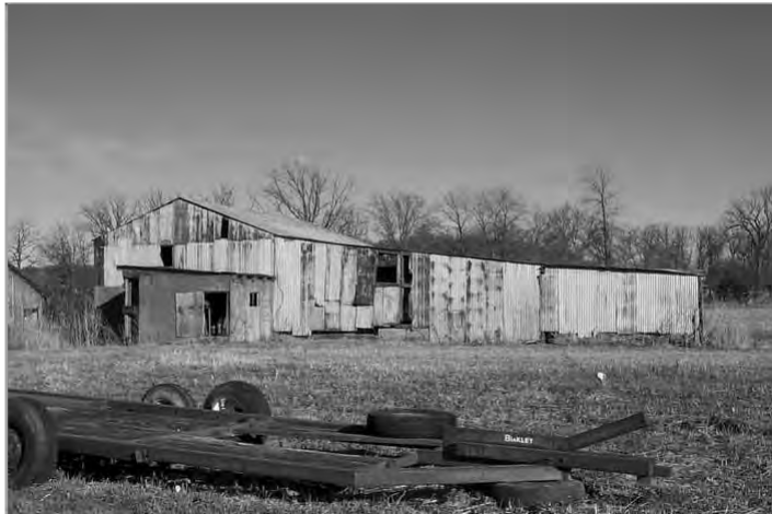
The structure illustrated at left is located on the Kobliski-Trantina farmstead in Section 8 of Homer Township. While it may not be aesthetically pleasing, it demonstrates the flexibility of configurations possible with pole barn structures.
