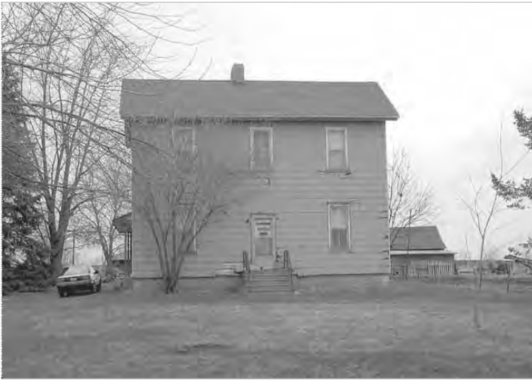
The Van Duser-Gooding-Peck-Weir-Cagwin farmstead was extant at the time of survey, but given the residential development in progress at the time of survey on the adjacent land it may be at risk for demolition. The Four-over-Four farmhouse is clad with asphalt shingle siding, a material homeowners turned to before artificial siding became available, and is set on a limestone foundation. The aerial view at upper left was taken in the early 1950s (This is Will County, Illinois, The American Aerial County History Series , No. 26 (1955)).
