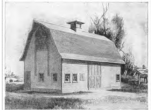
SMALL GENERAL FARM BARN OF NEAT DESIGN Size 46 by 28 feet. Ground floor stables four horses and three cows. Hay is put in through counterbalanced vertical sliding door. We can furnish complete set of blue-printed working plans and typewritten specifications for only $5.00 per set. When ordering, ask for Design No. A230L.
