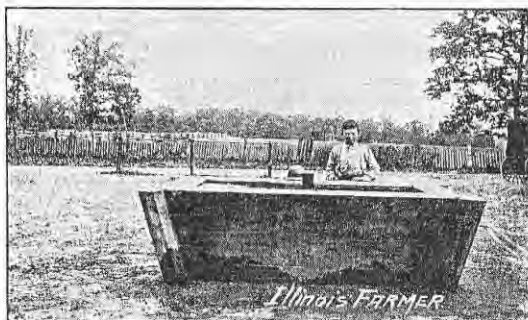
Concrete Stock Tank—8x4x3 feet. Cost $15.00
