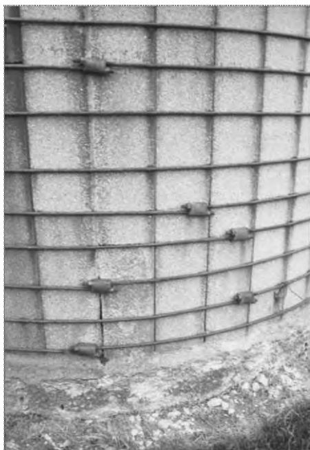
Detail views of the steel hoops and turnbuckles on a concrete stave silo.
