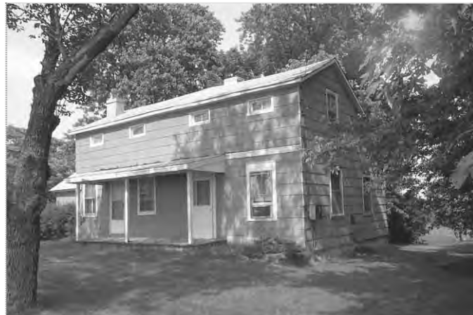
At left is the Davis-Corwin-Jungels-Beaver-De Pra farmhouse in Section 21 of Homer Township, which has had several additions; however, the original portion of the house was likely a Hall and Parlor structure.
