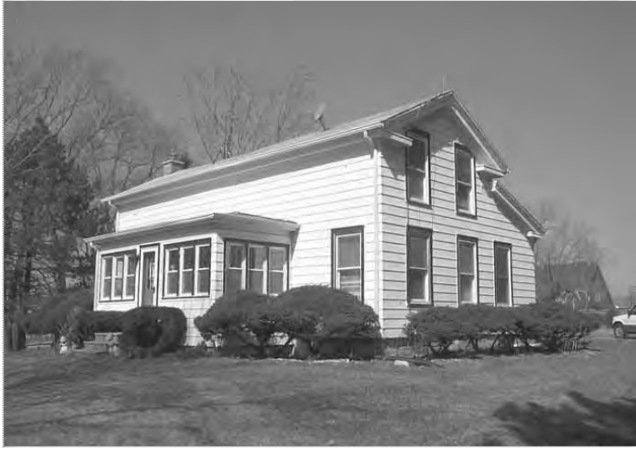
The farmhouse of the Brooks–Paddock–Hallis farmstead is the only historically significant element on the site. Despite the installation of artificial siding, and the possible eradication of small half-windows on the second floor of the main facade, the house retains its general appearance, including the Greek Revival detail at the gable ends.
