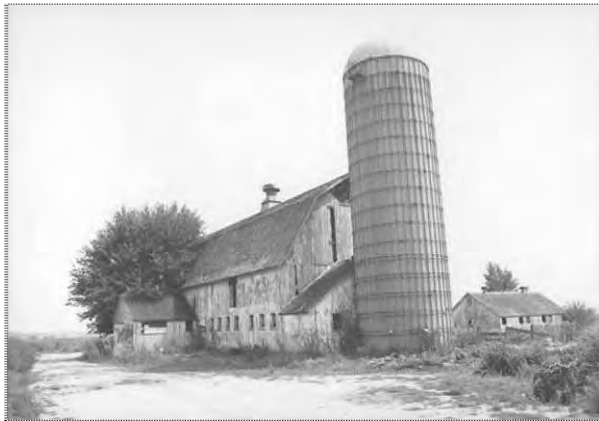
A Mason & Lawrence precast concrete stave silo is located on the site of the Haag farmstead in Section 18 of Wheatland Township. Although the other farm buildings on the abandoned site were demolished in early 2000, the silo was still standing in June 2002.
