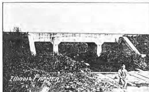
Concrete Bridge Across Drainage Ditch in Lawrence County, Illinois
