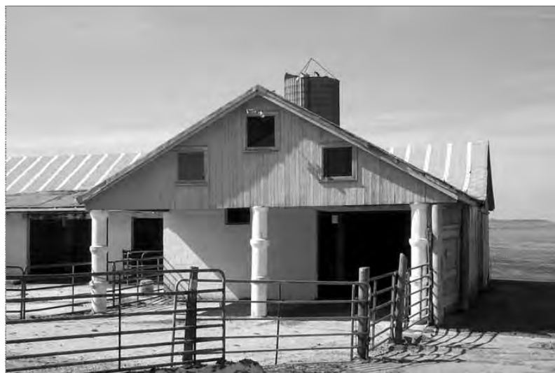
The Lucas-Gee farmstead in Section 15 of Homer Township has a horse barn that uses concrete pipe in a unique way. As shown in this detail view at left of a gable end, the structure has a sheltered porch reminiscent of a temple front.
