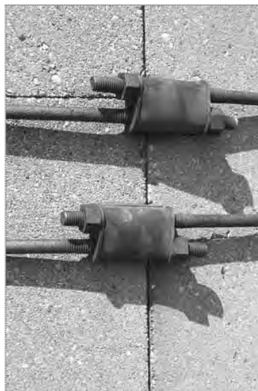
Detail views of the steel hoops and turnbuckles on a concrete stave silo.
