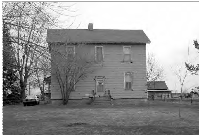
Shown above is the farmhouse on the Van Duser–Gooding–Peck–Weir–Cagwin farmstead in Section 31 of Homer Township.
