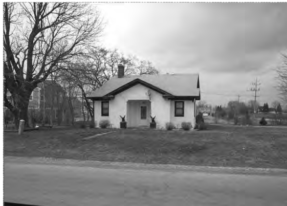
Shown at left is the former Barnett School at the northwest corner Gougar and Bruce Roads in Homer Township. The projecting eaves, the use of stucco, and overall bungalow form shows the influence of the Arts and Crafts Style.
