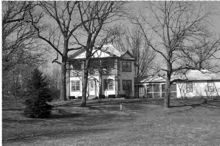
The house above was constructed by Akin Gorham in the 1860s. Located in Section 23 of Homer Township, subsequent owners probably added the pilasters and pediment facade to give what was originally a Victorian-era Italianate farmhouse a Georgian Revival appearance.
