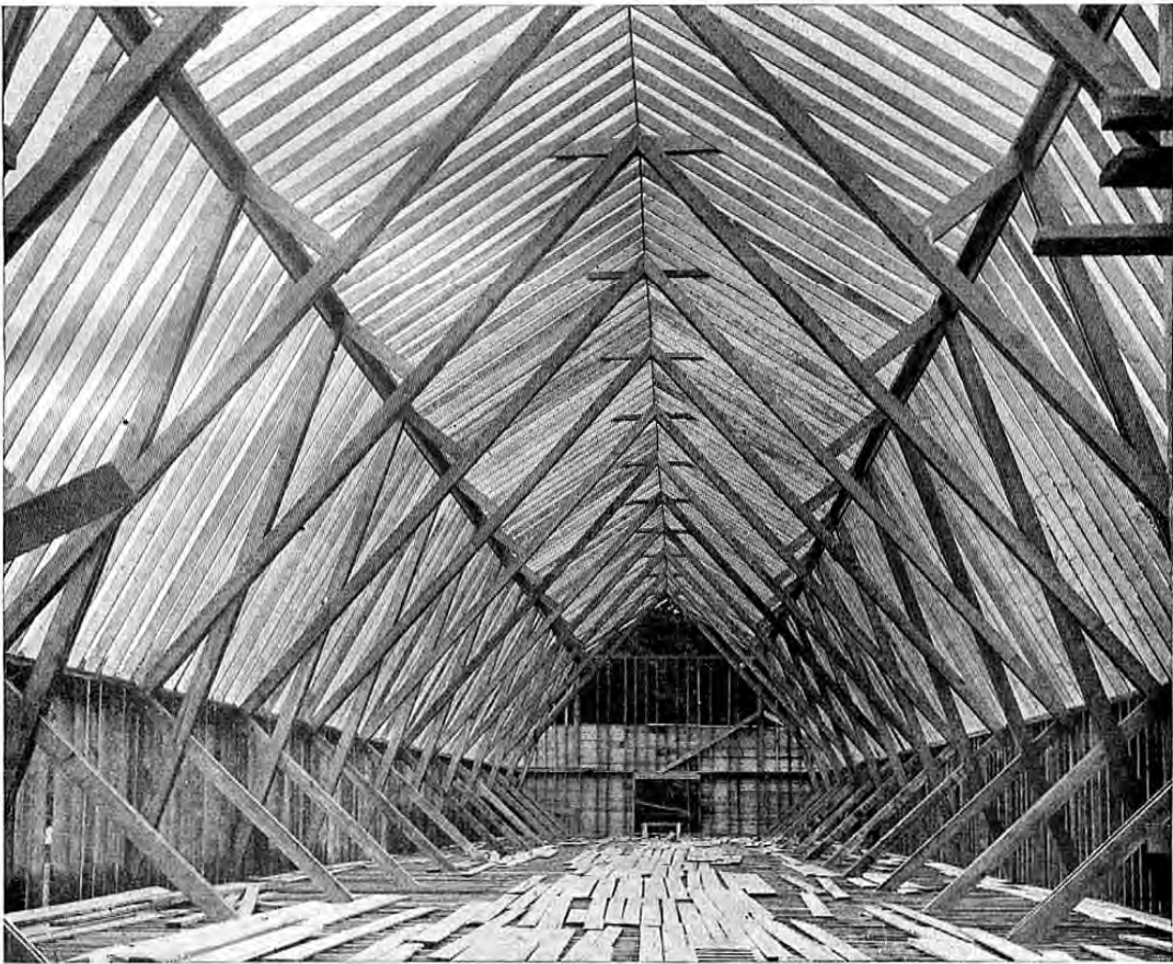
Another Type of Plank Frame Construction Self-Supporting Roof. A Truss is Placed Every 12 Feet, Membering at Four Points—Sill, Plate, Purlin and Ridge. Extra Bracing from the Sill out onto the Barn Floor is a Special Feature Giving Extra Strength. Notice Also How Purlin Plate is Built Up out of Two Timbers Laid Together at Right-Angles.
