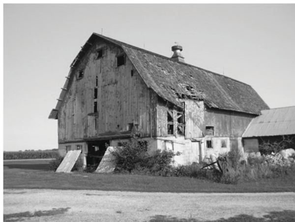
The survey area includes a number of concrete block structures. Above left: The historic concrete masonry farmhouse at the Clarence Cann Farmstead, site 1702, is built of concrete masonry. Above right: A detail of the rock-face concrete masonry units. Below left: The dairy barn at the Schroeder Farmstead, site 2206, has concrete block walls at the ground floor. Below right: The barn at the Smith–Von Alven Farmstead, site 3602, also uses concrete masonry for the first level.
