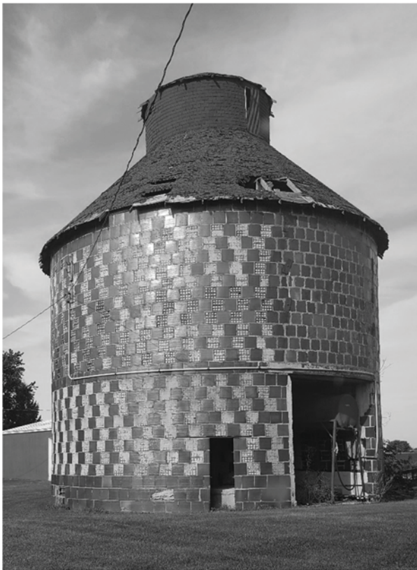
There are several distinctive perforated masonry crib barns in Will Township. Left: the circular crib barn at the Williams–Loitz Farmstead, site 3002. Right: The oblong crib barn at the Smith–Von Alven Farmstead, site 3602.
