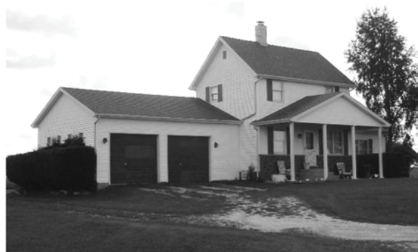
Left: The one-room deep original portion of the house at the Schroeder Farmstead, site 2206, is an example of the I House type. Right: The original two-story portion of the house at the Meyer-Sova Farmstead, site 2503, embodies the characteristics of the typical I House. (The one-story wings at right and left and the front porch are later additions.)
