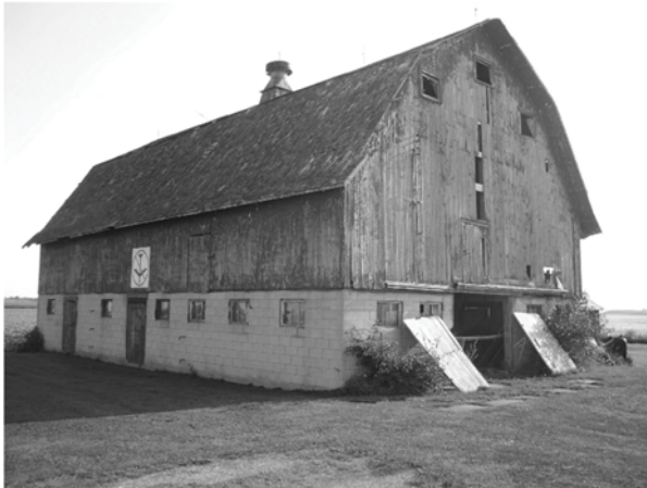
The Wisconsin Dairy Barn type is somewhat common in Will Township. Above left: The barn at the Nurberry–Szudarski Farmstead, site 405. This barn has an attached milk house. Above right: The barn at the Havens–Krumwiede Farmstead, site 602, is a typical example with ground floor stalls and an upper level hayloft. Below left: The barn at the Schroeder Farmstead, site 2206, is a later example with a ground floor of concrete masonry and an upper level constructed of wood framing. Below right: The barn at the Matthias–Koehn Farmstead, site 3605, is a particularly large and elaborate example.
