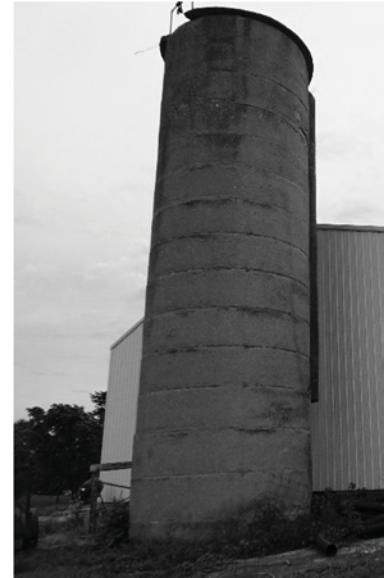
Left: The silo at the Bruns–Arnold Farmstead, site 101, is a typical example of a concrete stave silo in the survey area. Middle: The silo at the Kopman–DeYoung Farmstead, site 204, is a larger concrete stave example. Right: The silo at the Tong–Bate Farmstead, site 1801, is a relatively uncommon example of a cast-in-place concrete silo.
