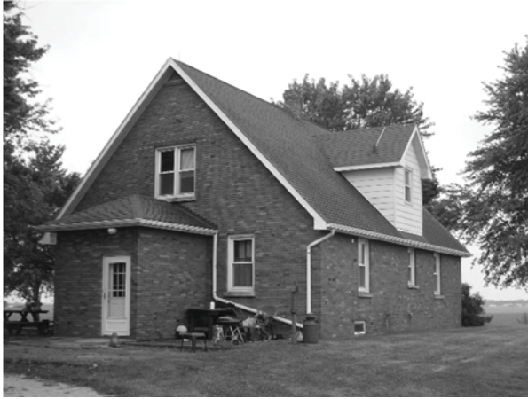
Left: The Cape Cod-type house at the Mittag Tenant Farm, site 2002, is constructed of brick masonry. Right: The well house at the Tong-Bate Farmstead, site 1801, is another local example of brick masonry construction.
