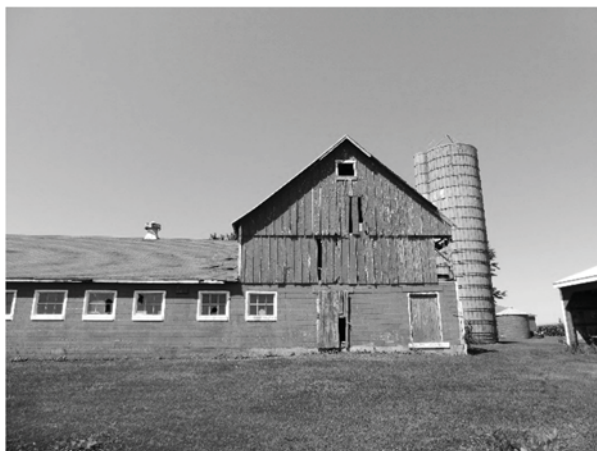
The survey area includes a number of concrete block structures. Above left: The historic concrete masonry farmhouse at the Clarence Cann Farmstead, site 1702, is built of concrete masonry. Above right: A detail of the rock-face concrete masonry units. Below left: The dairy barn at the Schroeder Farmstead, site 2206, has concrete block walls at the ground floor. Below right: The barn at the Smith–Von Alven Farmstead, site 3602, also uses concrete masonry for the first level.
