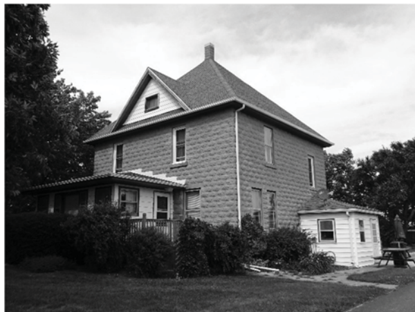
The survey area includes a number of concrete block structures. Above left: The historic concrete masonry farmhouse at the Clarence Cann Farmstead, site 1702, is built of concrete masonry. Above right: A detail of the rock-face concrete masonry units. Below left: The dairy barn at the Schroeder Farmstead, site 2206, has concrete block walls at the ground floor. Below right: The barn at the Smith–Von Alven Farmstead, site 3602, also uses concrete masonry for the first level.
