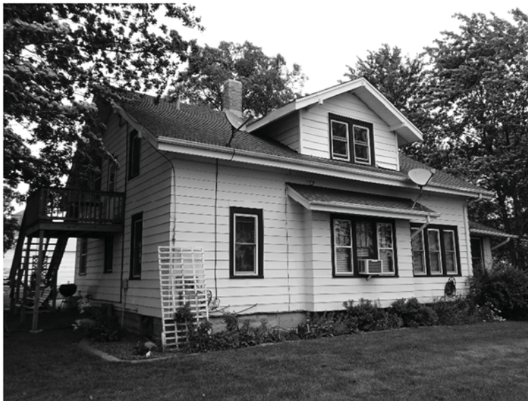
The bungalow at the Tong–Bate Farmstead, site 1801, shows Craftsman-inspired details such as three-over-one double-hung windows and Craftsman-style eave brackets.
