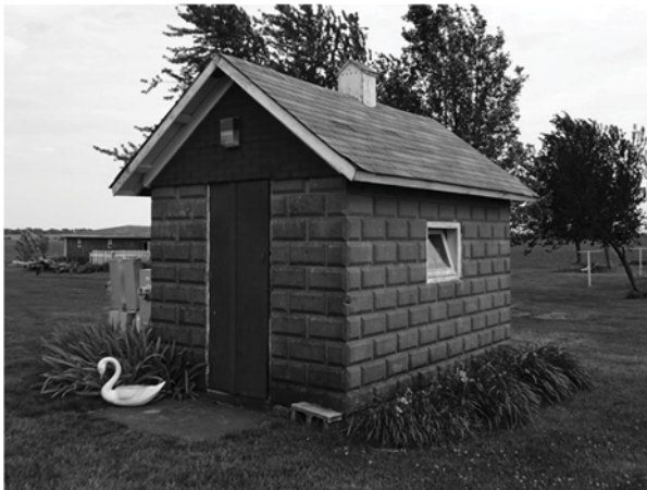
Many farmsteads have stand-alone well houses containing water pumping equipment. Left: The concrete masonry well house at the Clarence Cann Farmstead, site 1702. Right: The wood-framed well house at the Buhr–Hameister Farmstead, site 2402, is adjacent to an abandoned windmill.
