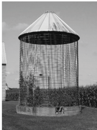
Above: Illustrations of two types of metal corn bins from The Illinois Farmer's Guide, August 1939. Below left: The grain bin at the Wilke Farmstead, site 704, is a typical early example of grain bin construction. Below middle: The mesh grain bin at the Stahlhuth-Seitz-Rauch Farmstead, site 2404, is a typical example of this 1950s type of construction. Below right: The three bins at the Loitz-Heisner Farmstead, site 1501, were built in the 1980s and are typical of new grain bin construction in the survey area.
