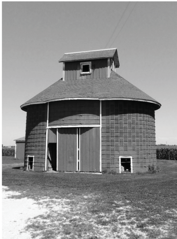
There are several distinctive perforated masonry crib barns in Will Township. Left: the circular crib barn at the Williams–Loitz Farmstead, site 3002. Right: The oblong crib barn at the Smith–Von Alven Farmstead, site 3602.
