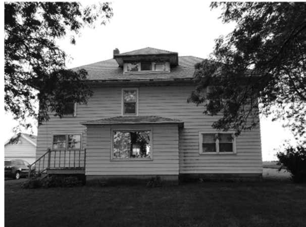
The American Foursquare type is common in Will Township. Left: The house at the Maves Farmstead, site 1601, includes a pyramidal roof, hipped dormer, symmetrical plan, and front entrance porch characteristic of the American Foursquare building type. Right: The house at the Conrad–Cann Farmstead, site 1803, is also a local example of the building type.
