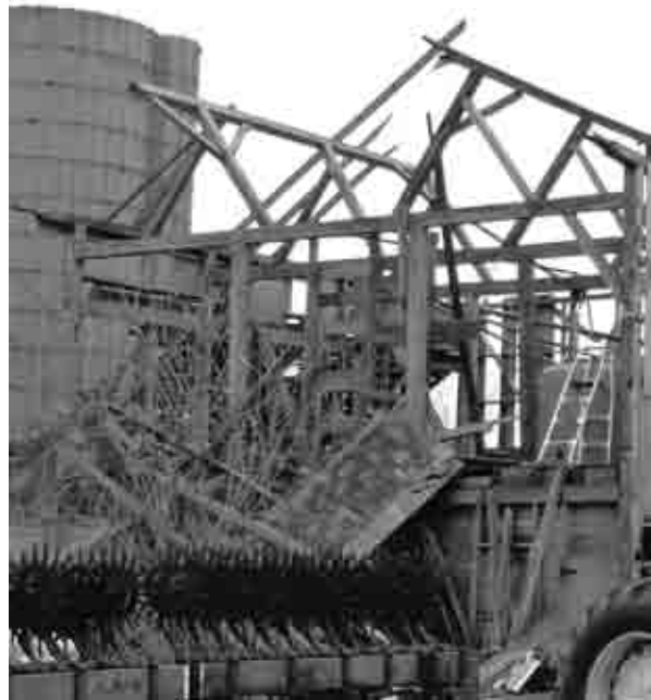
Left: A drawing of heavy timber barn framing from 1894 [William E. Bell, Carpentry Made Easy, or the Science and Art of Framing (Philadelphia: Ferguson Bros. & Co., 1894), plate 7]. Right: This type of braced heavy timber framing is visible in the partially dismantled barn at the Rogers–Denning Farmstead in Section 18 of Peotone Township.
