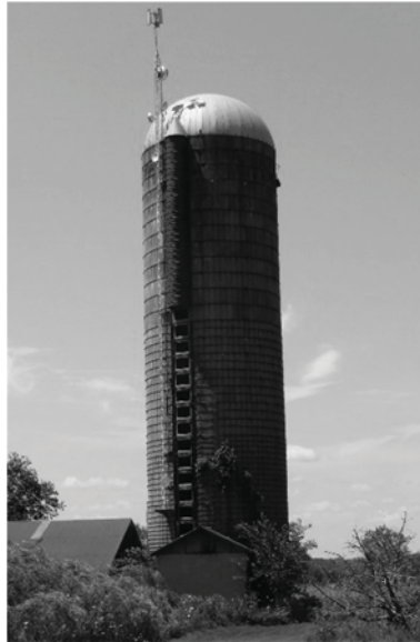
Left: The silo at the Bruns–Arnold Farmstead, site 101, is a typical example of a concrete stave silo in the survey area. Middle: The silo at the Kopman–DeYoung Farmstead, site 204, is a larger concrete stave example. Right: The silo at the Tong–Bate Farmstead, site 1801, is a relatively uncommon example of a cast-in-place concrete silo.
