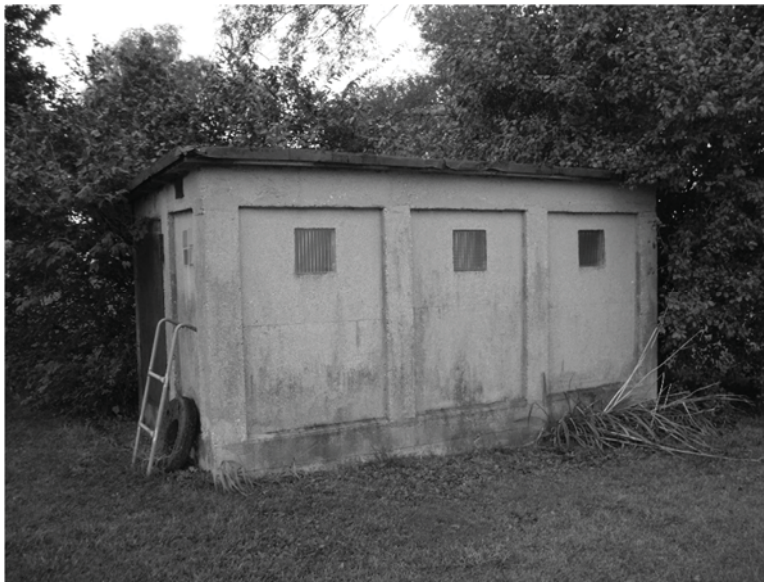
This cast-in-place concrete storage building, likely dating to the 1940s, is at the Havens–Krumwiede Farmstead, site 602.
