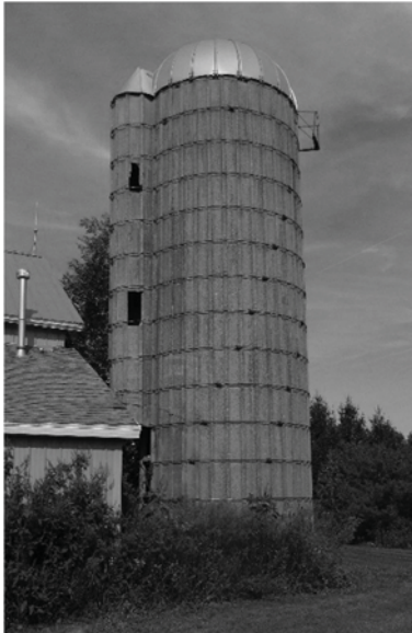
Left: The silo at the Bruns–Arnold Farmstead, site 101, is a typical example of a concrete stave silo in the survey area. Middle: The silo at the Kopman–DeYoung Farmstead, site 204, is a larger concrete stave example. Right: The silo at the Tong–Bate Farmstead, site 1801, is a relatively uncommon example of a cast-in-place concrete silo.
