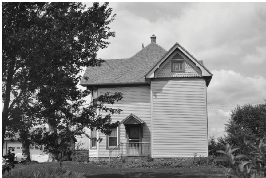
What style is it? The house at the Hagenow Farmstead, site 703, retains some Queen Anne style details, but the original character of this nineteenth century house has been obscured by the closing up of most of the street-facing windows.
