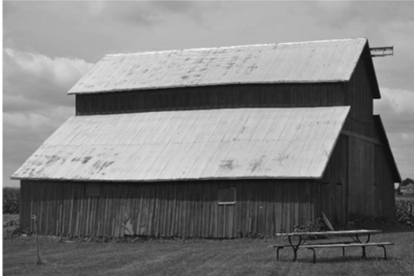
The barns at the Hagenow Farmstead, site 703 (left) and the Smith–Von Alven Farmstead, site 3602 (right) are examples of the Feeder Barn type.
