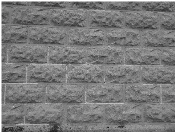
The survey area includes a number of concrete block structures. Above left: The historic concrete masonry farmhouse at the Clarence Cann Farmstead, site 1702, is built of concrete masonry. Above right: A detail of the rock-face concrete masonry units. Below left: The dairy barn at the Schroeder Farmstead, site 2206, has concrete block walls at the ground floor. Below right: The barn at the Smith–Von Alven Farmstead, site 3602, also uses concrete masonry for the first level.
