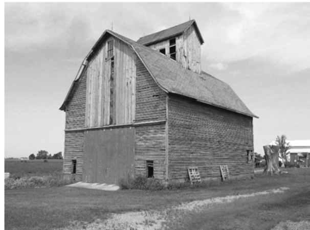
There are many wood crib barns in Will Township. Examples differ in size, roof shape, materials, and the presence of a cupola for the grain elevator equipment. Illustrated here, examples of crib barns include: above left, early crib barn at the Hagenow Farmstead, site 703; above right, early crib barn at the Matthias Farmstead, site 2302; below left, crib barn with elaborate elevator housing and cupola at the Bunte Farmstead, site 3603; and below right, a typical gambrel roof crib barn from the 1920s–1940s era, at the Thiede–Bunte Farmstead, site 2205.
