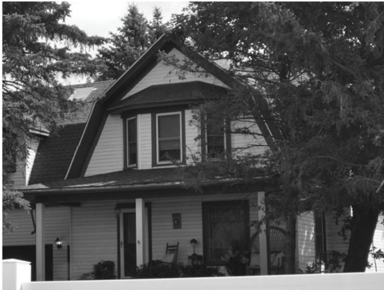
The house at the Felton–Mundt Farmstead, site 1804, has a front-facing gambrel-roof shape and leaded art glass windows, referencing the Dutch Colonial Revival style.
