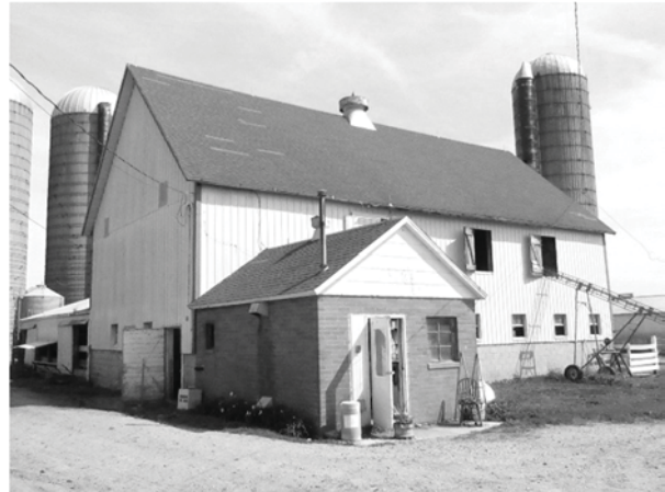
The Wisconsin Dairy Barn type is somewhat common in Will Township. Above left: The barn at the Nurberry–Szudarski Farmstead, site 405. This barn has an attached milk house. Above right: The barn at the Havens–Krumwiede Farmstead, site 602, is a typical example with ground floor stalls and an upper level hayloft. Below left: The barn at the Schroeder Farmstead, site 2206, is a later example with a ground floor of concrete masonry and an upper level constructed of wood framing. Below right: The barn at the Matthias–Koehn Farmstead, site 3605, is a particularly large and elaborate example.
