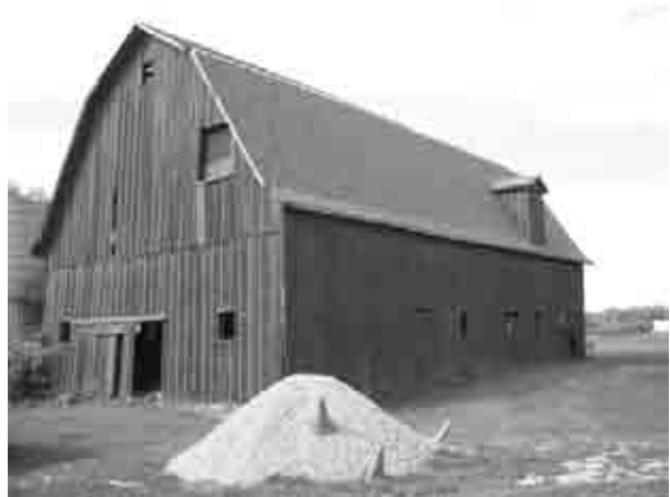
Examples of the plank frame barn type from Crete Township. Above left: Bruns Farmstead, site 7902. Above right: The Bruns–Rehborg Farmstead, site 7901. Lower left: A gambrel rood plank frame barn at the Hartman–Koelling Farmstead, site 2504. Lower right: An example of the plank frame barn type illustrated in Smith & Betts Farm and Building Book (Chicago: The Radford Architectural Company, 1915).
