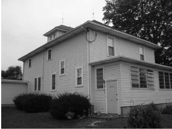
Above left: The house at the Gustave Ohlendorf Farmstead, site 3402, includes a pyramidal roof, hipped dormer, symmetrical plan, and front entrance porch characteristic of the American Foursquare building type. Above right: The Kraegel–Langebartels Farmstead, site 3205, is also a local example of the building type. Below: The American Foursquare house at the Hartman–Koelling Farmstead, site 2504, features a hipped dormer as well as a distinctive front porch design.
