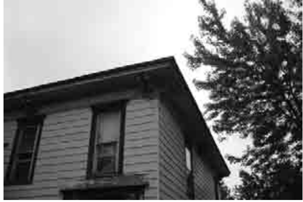
Left: The house at the Heller-Krol Farmstead, site 3301, features a low pitched hip roof with overhanging eaves and a bracketed Italianate style cornice. Right: A detail of the overhanging eaves and bracket cornice at the house at the Heller-Krol Farmstead.
