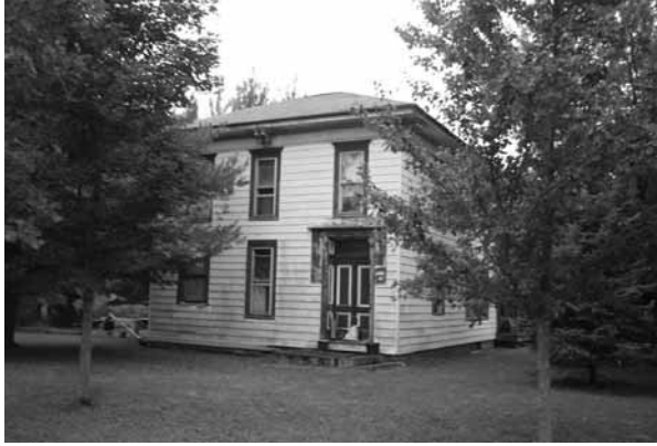
Left: The house at the Heller-Krol Farmstead, site 3301, features a low pitched hip roof with overhanging eaves and a bracketed Italianate style cornice. Right: A detail of the overhanging eaves and bracket cornice at the house at the Heller-Krol Farmstead.
