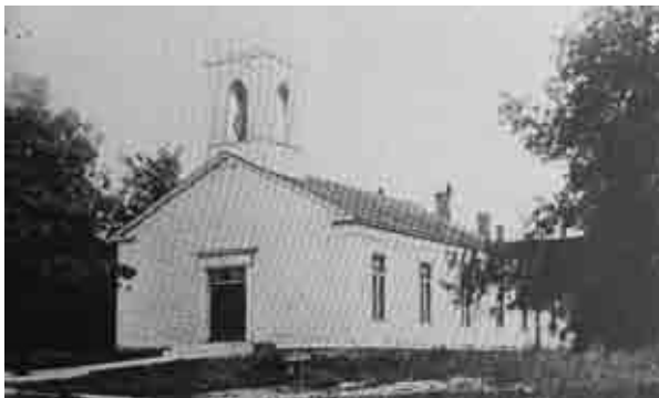
Left: First Congregational Church of Crete, constructed in the 1850s, photo after the loss of the original steeple in 1900.
