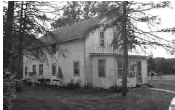
Left: The circa 1889 house at the Harmening–Parke Farmstead, site 1802, has a symmetrical massing typical of the Four-over-Four type (with later one-story additions to the sides). Right: The house at the Bremer–Meyer–Wolf Farmstead, site 5802, is an example of a Gable Front type structure.
