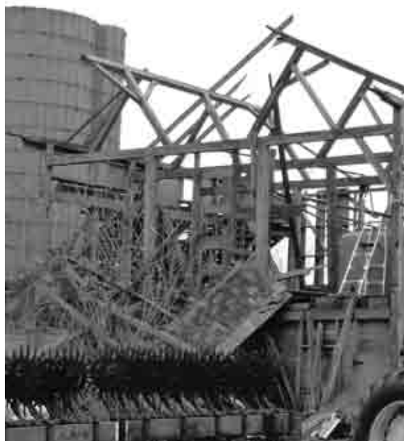
Left: A drawing of heavy timber barn framing from 1894 [William E. Bell, Carpentry Made Easy, or the Science and Art of Framing (Philadelphia: Ferguson Bros. & Co., 1894), plate 7]. Right: This type of braced heavy timber framing is visible in the partially dismantled barn at the Rogers–Denning Farmstead in Peotone Township.
